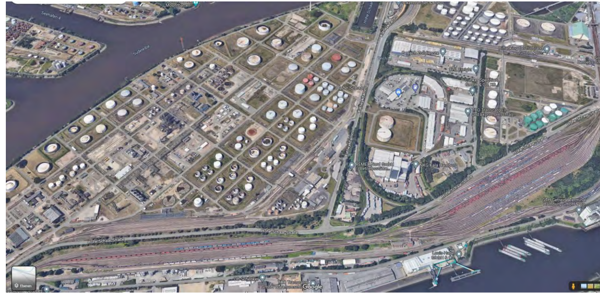
Railway track systems for the assembly of tank wagons in the Hamburg port.
